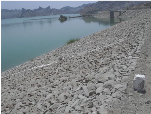
Upstream Face of Dam
