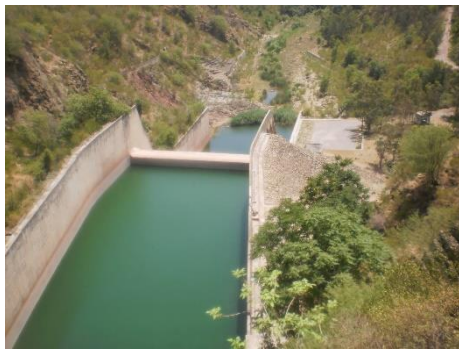
Spillway Stilling Basins
