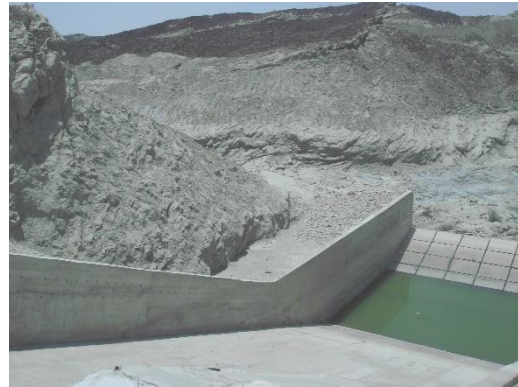
Main Spillway Flip Bucket
