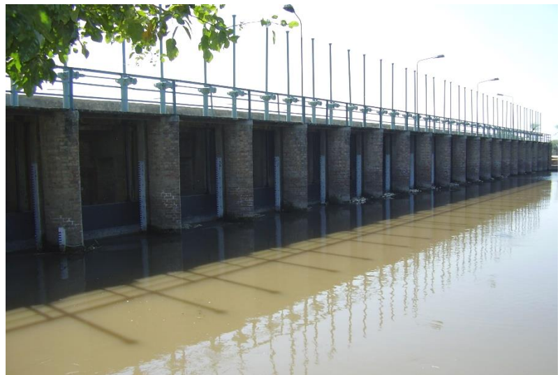
LBDC Fall Structure
