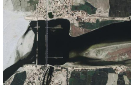
Aerial View of Existing Barrage
