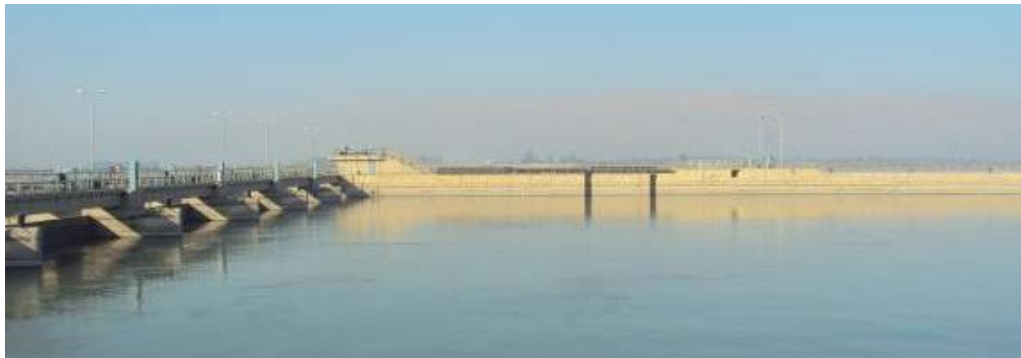
View Upstream of the Chashma Barrage
