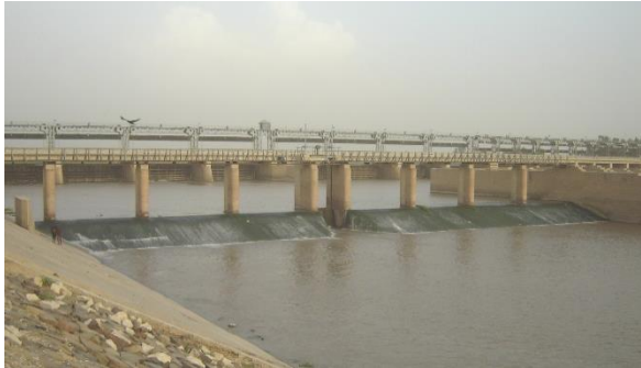
Islam Barrage - View from downstream side
